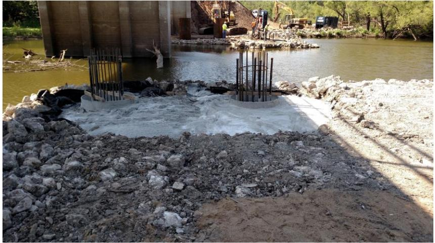
Proper containment of concrete slurry on a set of drilled shafts. How would you handle this situation?
