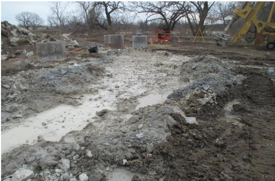
Drilled shafts with little to no controls in place to contain the concrete slurry and spoils from the operation.
